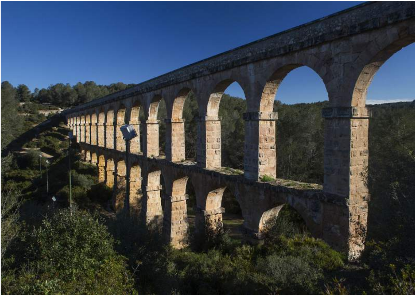
Les Ferreres Aqueduct / Pont del Diable Bridge (Devil's Bridge) © Manel Antolí (RV Edipress)
